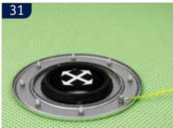
**(UK)** To establish weep holes and enable horizontal adjustment of the upper part, turn the sealing ring upside down.
