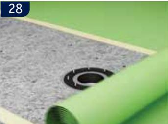
**(UK)** Install the (flat) sealing ring. Lay the sheet membrane in accordance with the guidelines from the supplier of the sheet membrane.
