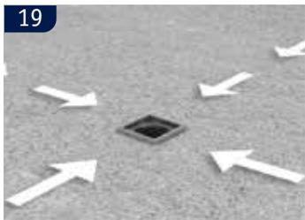
(UK) Cast the floor with the recommended fall towards the drain. For drains with 50 mm liquid membrane flange, a liquid membrane can be applied in accordance with the guidelines of the supplier of the liquid membrane
